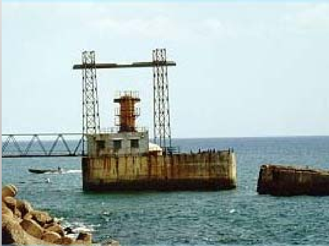
Indian Wave Power Plant at Vizhinjam
