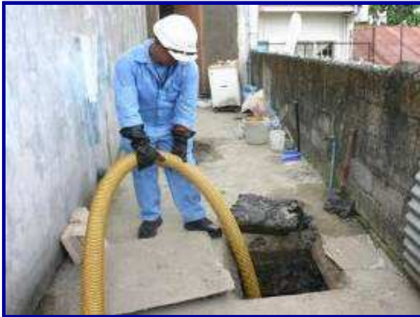
Septic Tank Desludging & Septage Treatment
