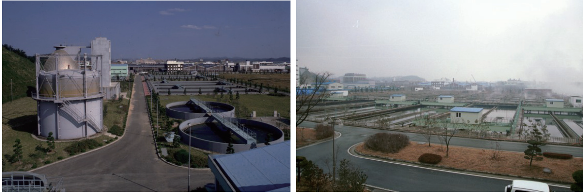
Ansan Wastewater Treatment facility (source: Ansan Internet News)
