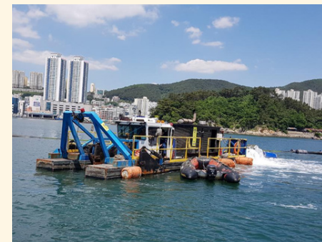
Operation of a sediment improvement project at Dadaepo port. Polluted sediments are dredged to a barge (right photo) to transport to land where sediments are properly treated and disposed of.
