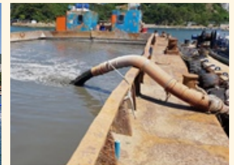
Operation of a sediment improvement project at Dadaepo port. Polluted sediments are dredged to a barge (right photo) to transport to land where sediments are properly treated and disposed of.
