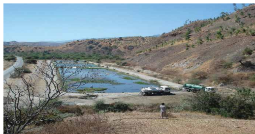
Wastewater treatment pond (Source: Carlos Ximenes, 2016)
