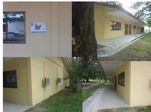
Dili Port offices.
