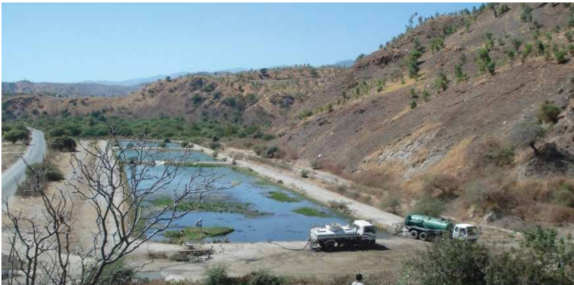
Figure 13.6: Wastewater Treatment Ponds in Tasitolu.
