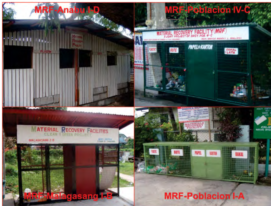
Materials recovery facilities in Imus (2007).
