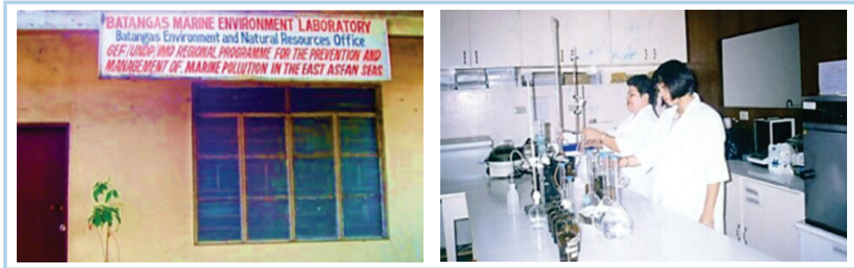
Figure 1. The BEL building in 1998.
