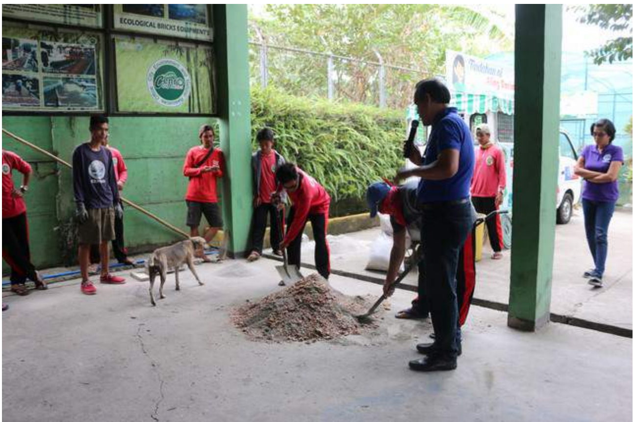
Hand-mixed ecobrick material
