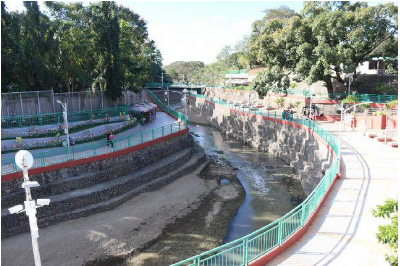
Promenade des Dasmariñas is still under construction
