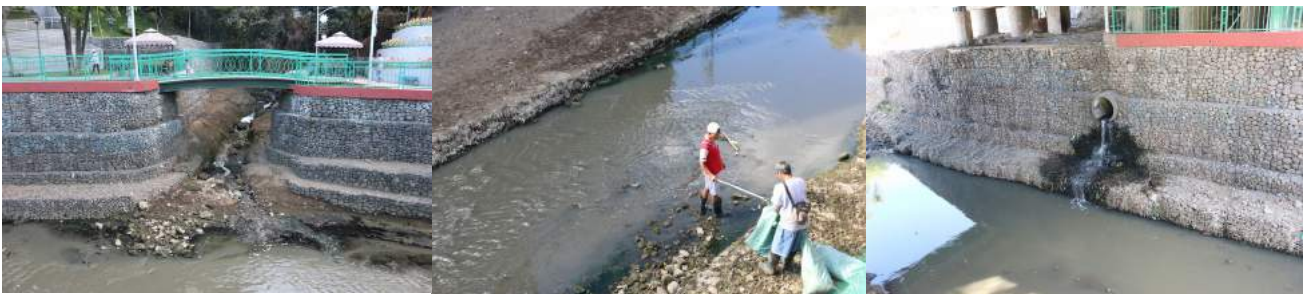
Small inlets, trash pickers, and a pipe flowing directly into the river which seems to have waste coming out of it
