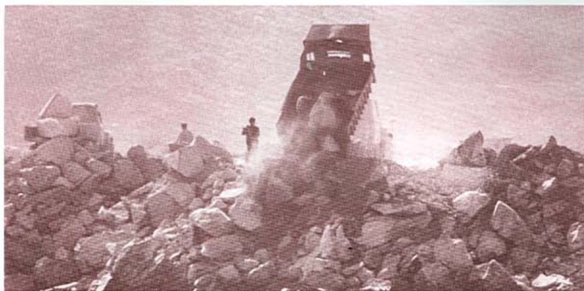
Coastal reclamation without cofferdam.
