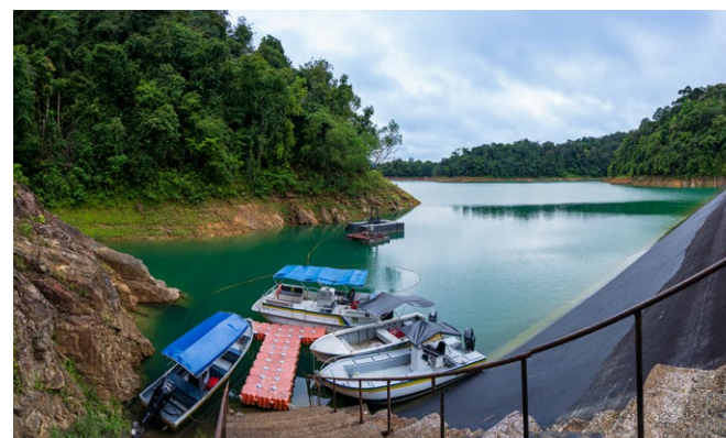
Boats anchored along the edge of Pedu Dam, one of the main reservoirs supplying water to the Kedah River Basin. Surrounded by forested catchments, the dam plays a critical role in water supply, flood regulation, and downstream irrigation. (Photo by Orange Omengan/PEMSEA)
